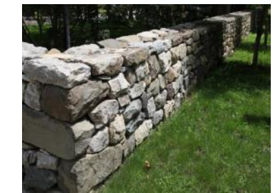
Dry Stack Stone Wall
