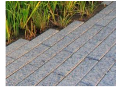
Linear Concrete Unit Paving
