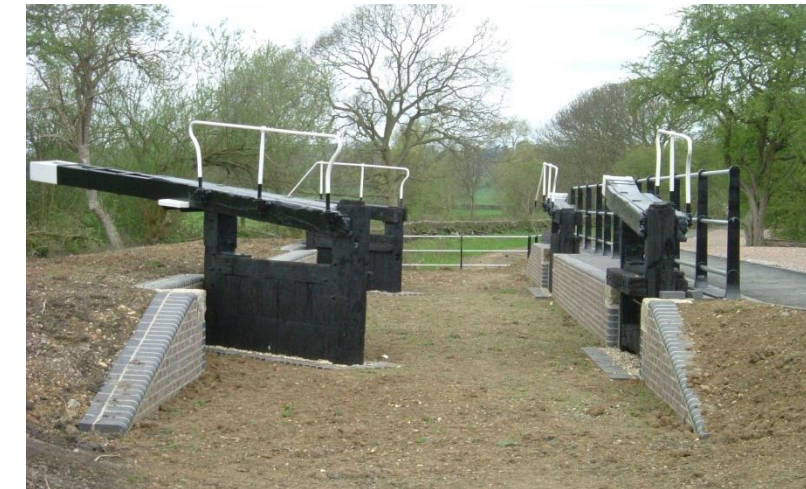
Figure 46 - Example of interpretive installation commemorating historic locks.
